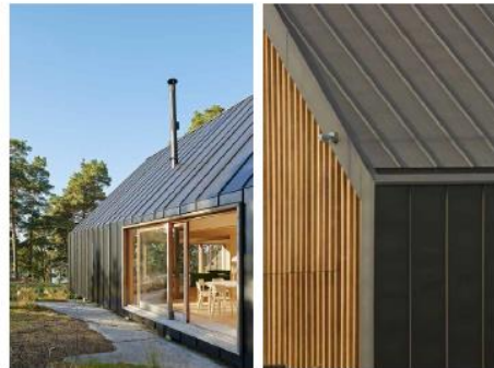
2. Zinc Standing Seam Roof
